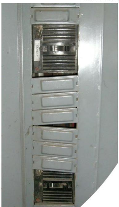
Breaker switches or blanks must be used to cover open breaker slots. Staggering or tape is not allowed. Photo below shows proper condition.
