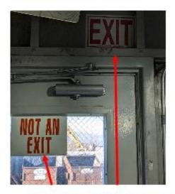
Not correct - Labeled both as "Exit" and "Not an Exit"
