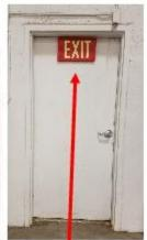
Not correct — Exit sign on door, not visible is door is open
