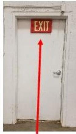
**Not correct – Exit sign on door, not visible is door is open**
