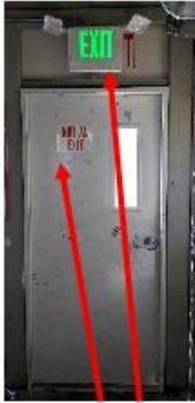
**Not Correct – Door marked as both "Exit" and "Not an Exit"**
